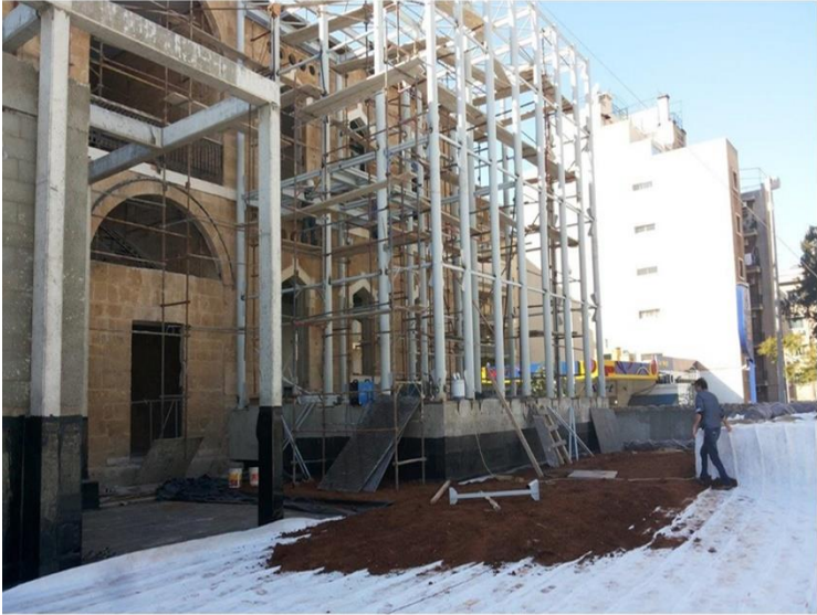
Beginning of the covering with soil.
