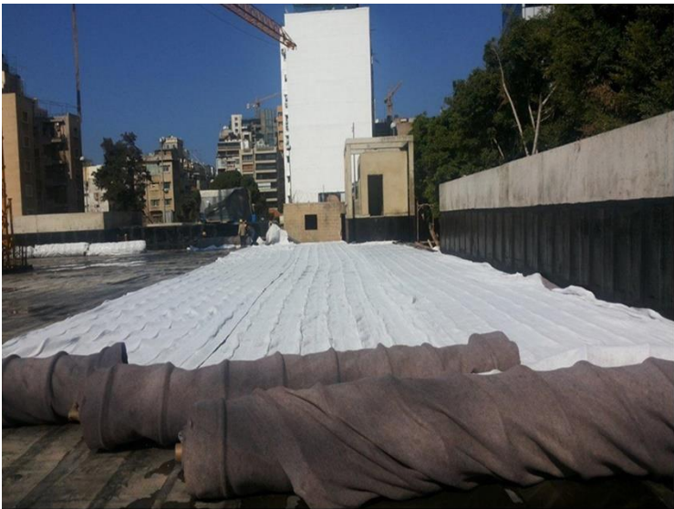
Start of installation of the product.
