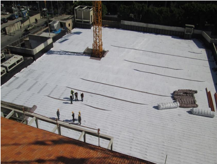
Overview of the construction site
